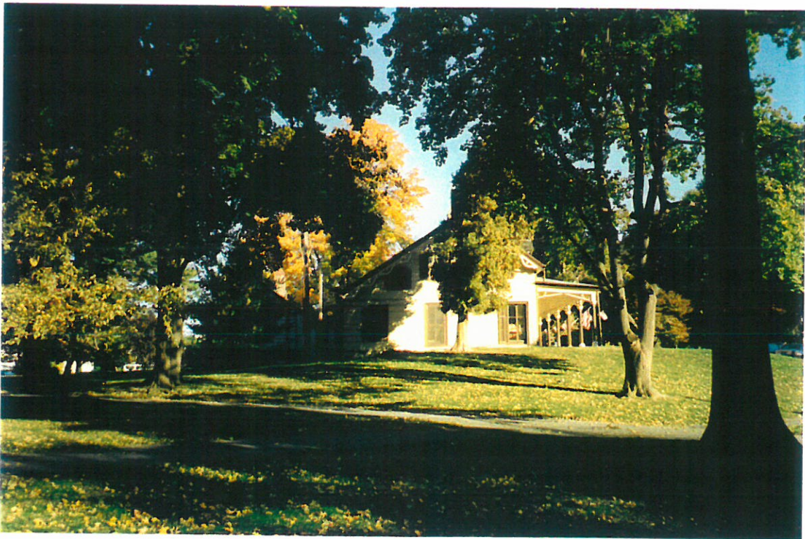
The Mesier Homestead - West Elevation
