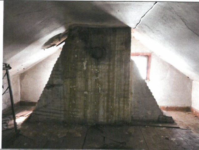
Photo 56. Area A, Room 203, modified chimney, looking east.
