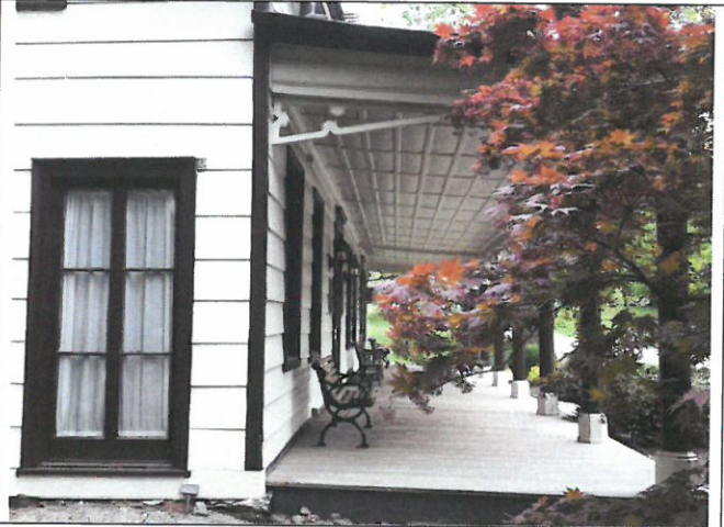
Photo 19. Porch looking east.
