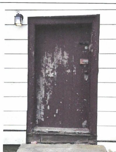
Photo 43. Area A, entrance door N11, north elevation.
