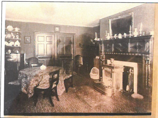
Photo 12. Room 112, looking northeast, c.1880s, (at Homestead).
