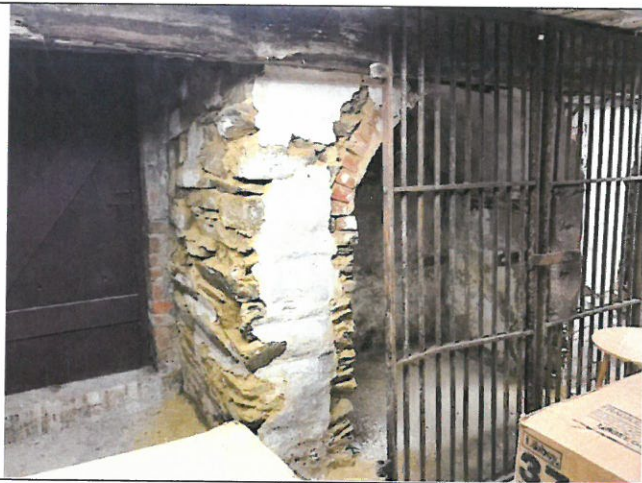
Photo 70. Area D, Room 002, Chimney A west face.
