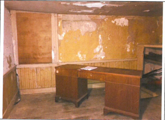
Photo 49. Area A, Room 101, looking south, window opening converted from original door.
