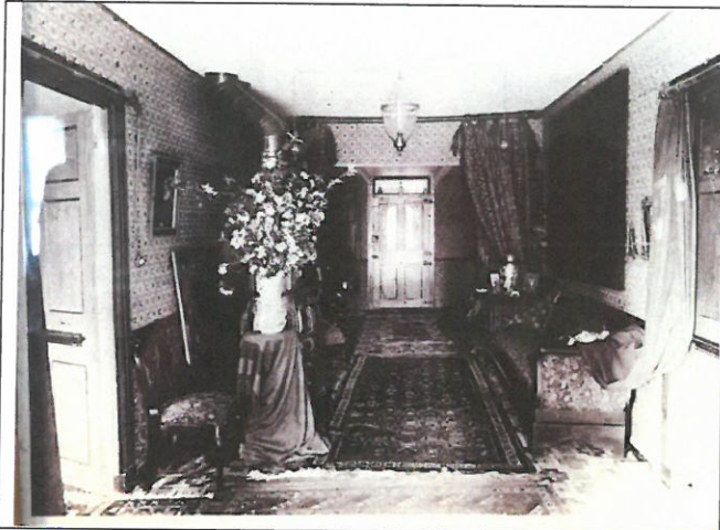
Photo 6. Room 106N, looking north, c.1880s, (at Homestead).
