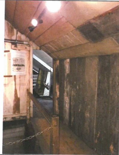
Photo 103. Area C, Stair 2, looking west.
