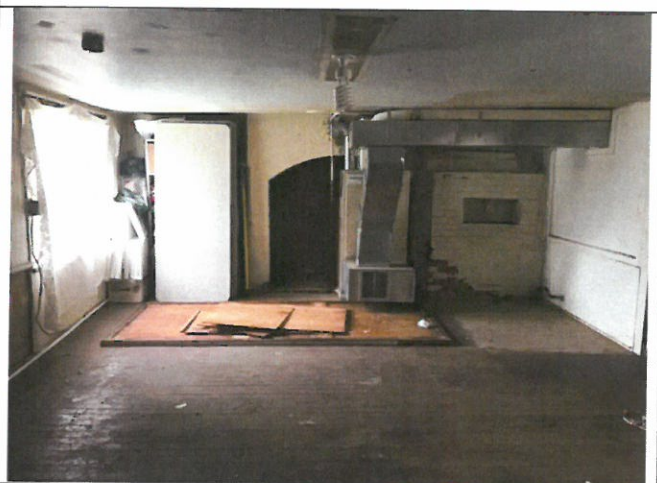
Photo 45. Area A, Room 102, looking east.
