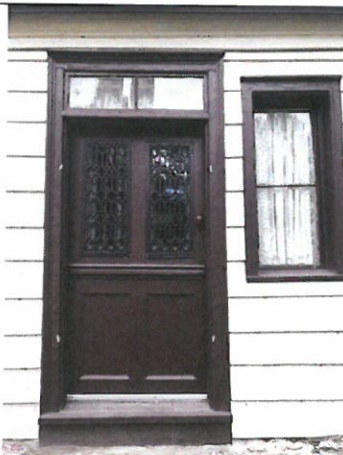
Photo 41. Area D, hall door N6, north elevation .
