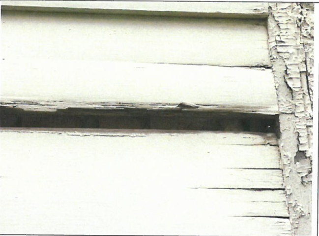
Photo 35. Siding and trim condition, typical.
