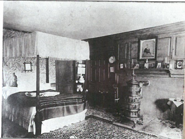
Photo 8. Room 113, looking northeast, c.1880s, (at Homestead).
