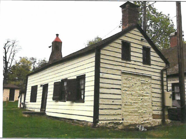
Photo 20. Area A, north and west elevations.
