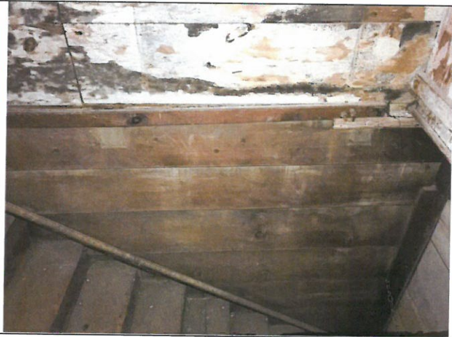
Photo 105. Area C, Stair 2, looking south. Original exterior framing and finishes visible.
