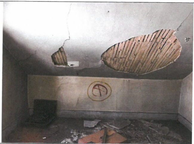
Photo 53. Area A, Room 201, looking north.
