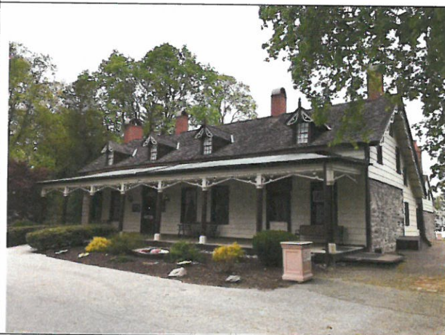
Photo 14. South and west elevations.
