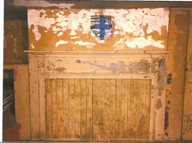
Photo 50. Area A, Room 101, west mantle/fireplace.
