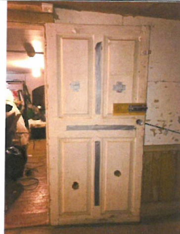
Photo 51. Area A, Room 102, original door with modifications.
