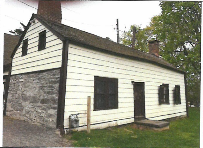
Photo 21. Area A, east and north elevations.
