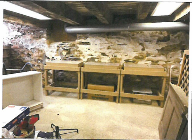
Photo 69. Area D, Room 002, south wall.
