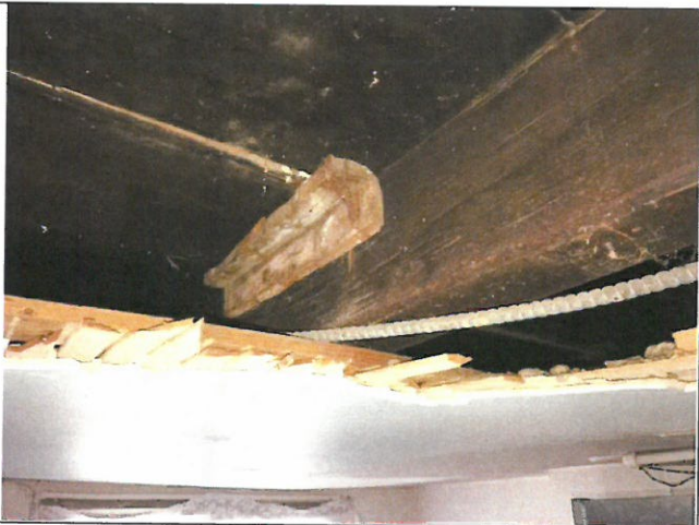
Photo 46. Area A, wood framing and trim above ceiling, Room 102.
