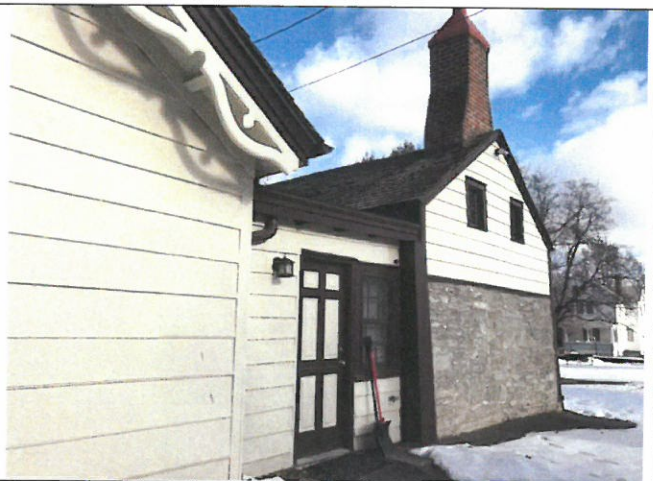
Photo 23. East elevation, from left: Areas C, B, A.
