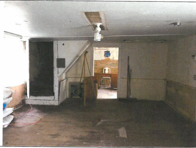
Photo 44. Area A, Room 102, looking west.
