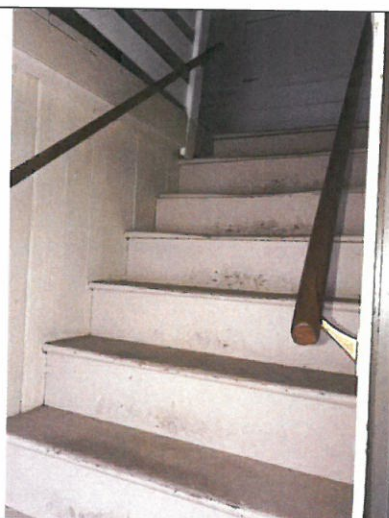
Photo 83. Area C, Stair 3, looking south.
