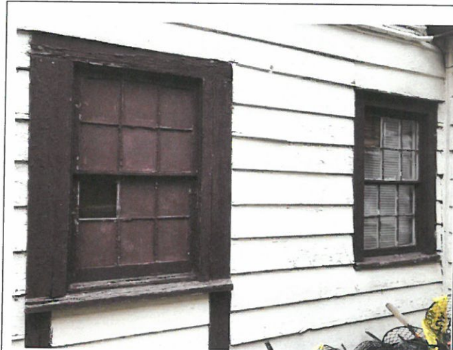
Photo 36. Area A, windows, south elevation.
