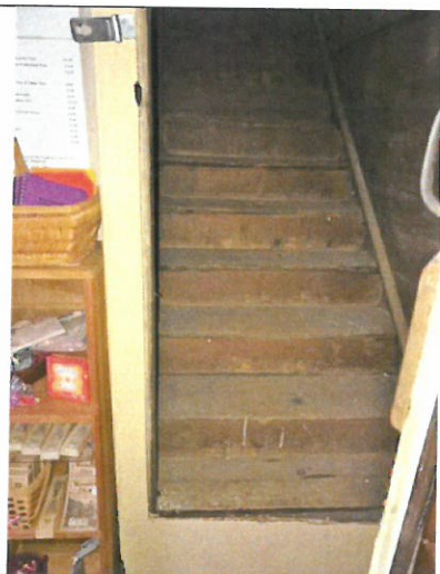
Photo 82. Area C, Stair 2, looking east.
