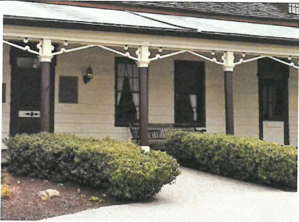
Photo 40. Area D, hall and entrance doors S7 and S10, south elevation.
