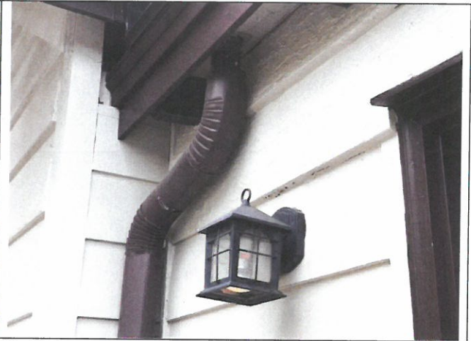
Photo 31. Area B, roof drainage.
