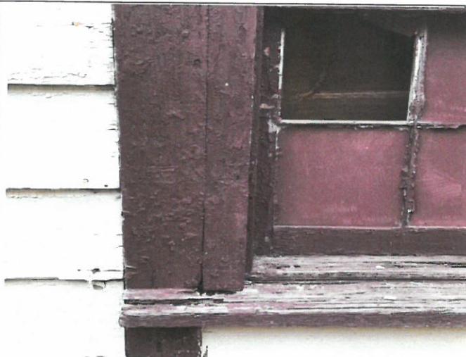
Photo 37. Area A, window, typical condition, windows and sills.
