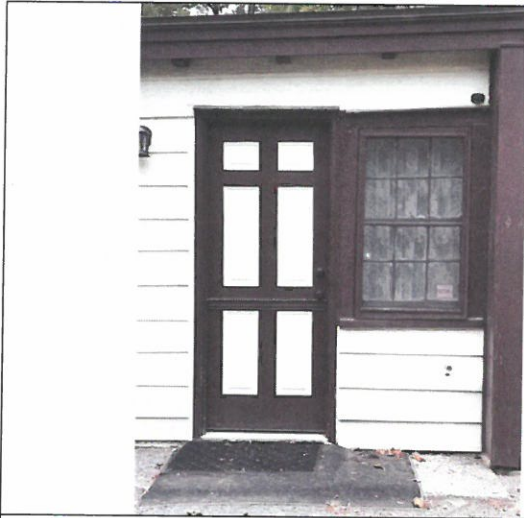
Photo 42. Area B, entrance door E7, east elevation.
