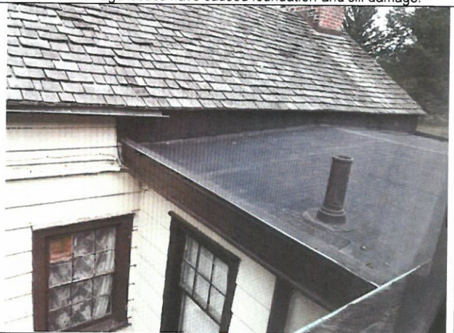
Photo 27. Area B, connector roof.
