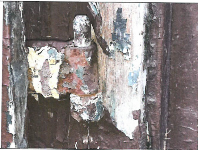
Photo 39. Area A, shutter hardware, detail.
