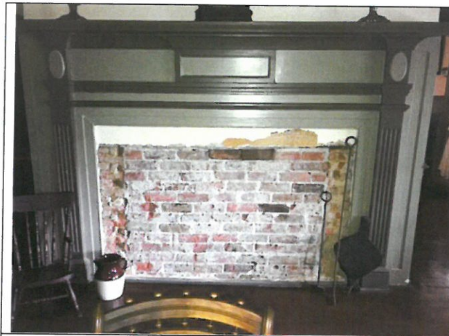
Photo 90. Area D, Room 112, fireplace detail.
