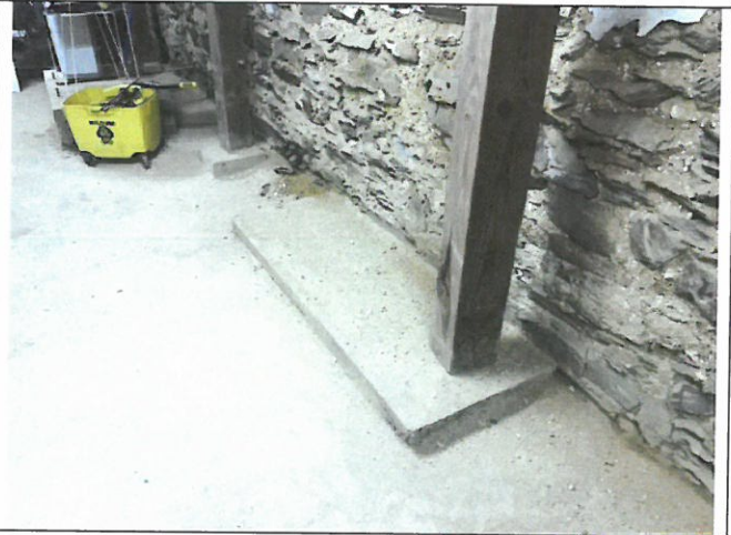
Photo 67. Area D, Room 001, north wall new posts and concrete slab.
