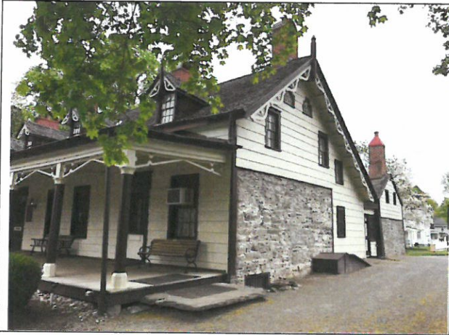
Photo 18. West elevation and porch (Area E).
