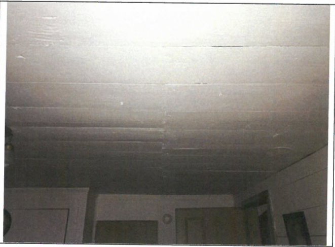
Photo 115. Area D, Room 211, looking north.
