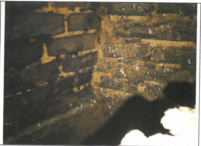
Photo 91. Area D, Room 112, view into fireplace (original construction visible).
