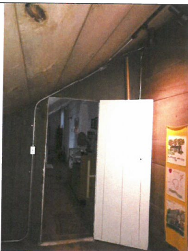
Photo 94. Area C, Room 204, looking east.
