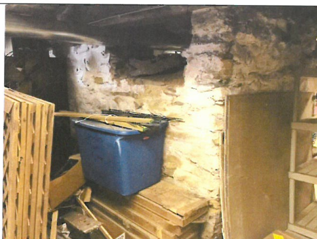
Photo 63. Area D, Room 001, Chimney B east face.
