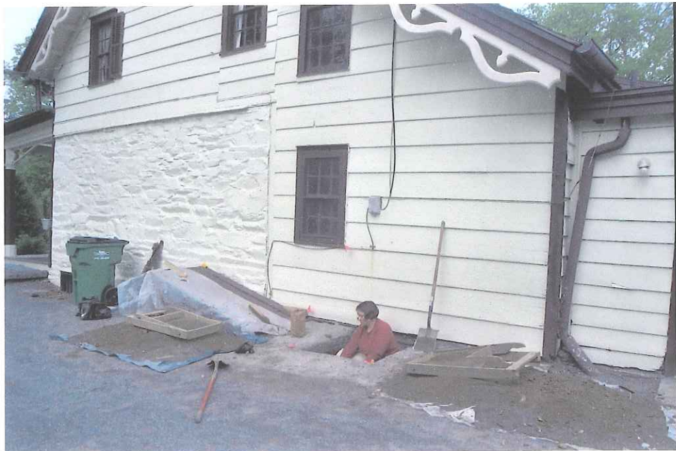
Figure 14: Archeologist working in Unit 5, placed on the southeast side of the larger 1750s Brewer-Mesier house. View facing west.
