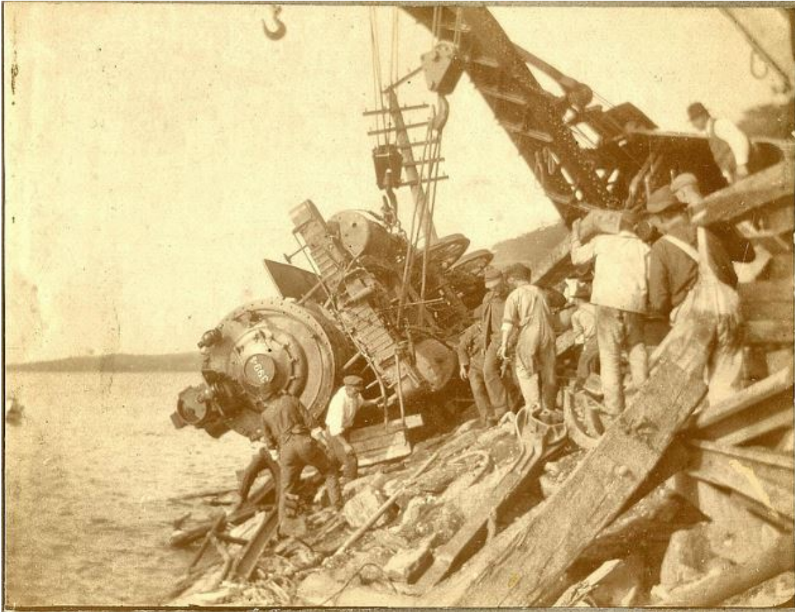
Photo of Wrecked Train Engine No. 3994
